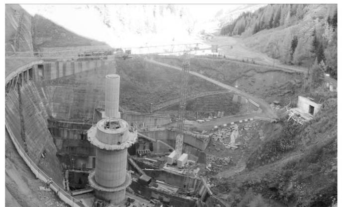
Figure 10: New structure at the downstream toe of the dam during construction
