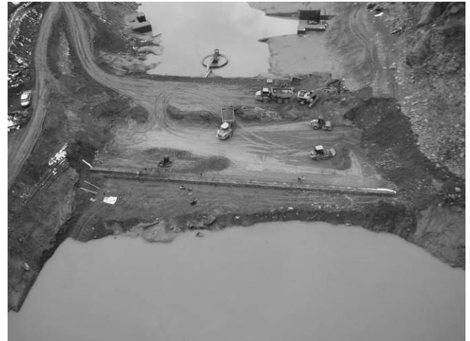
Figure 6: Excavations for new cofferdam construction
