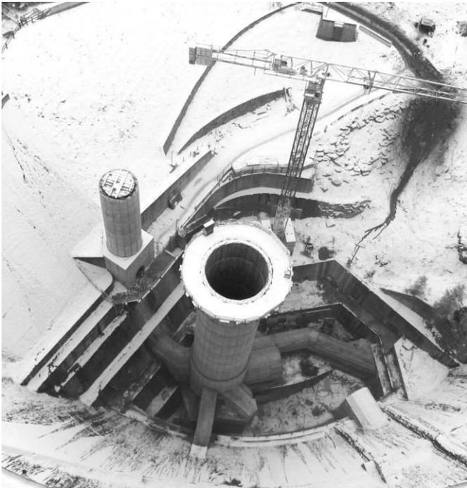
Figure 12: Inspection shafts
