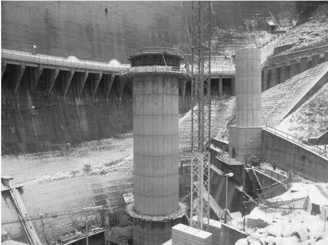
Figure 11: Main shaft during construction
