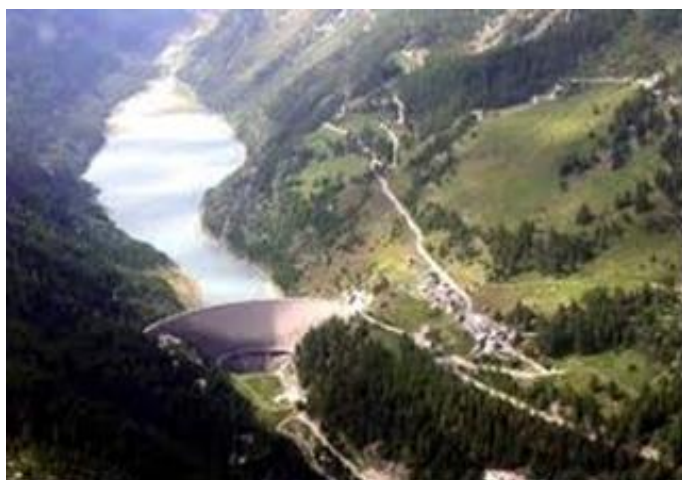
Figure 1. Aerial view of the dam located in the Valgrisenche Valley / Vista aerea della diga in Valgrisanche.
